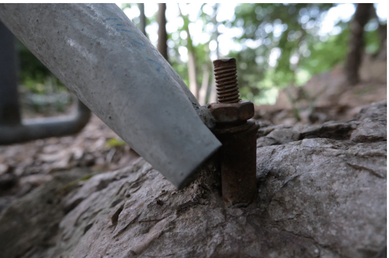
Relationship between steel tube, screw and stone
